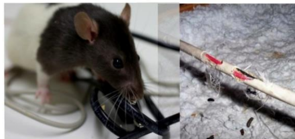
Rodent Chewing Cables
