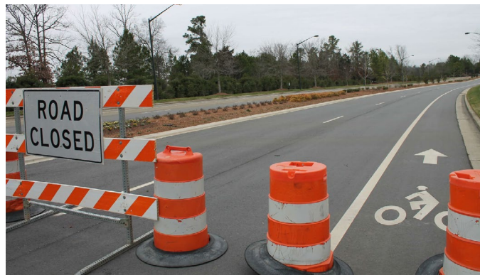
Fig. 13: Sign of transportation hazard
