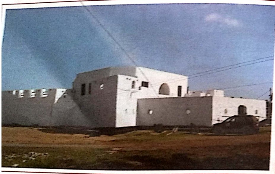
Fort Apollonia in Beyin (Western Region), built in 1768 by the British
