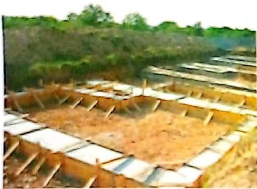
Clearing forest for housing
