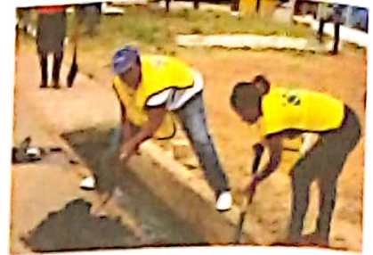
Cleaning the gutters
