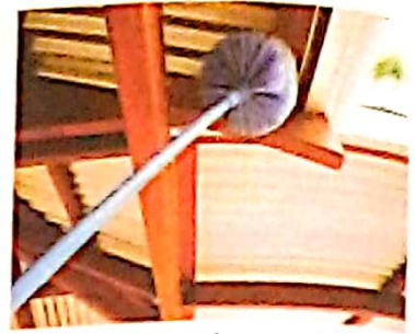
Cleaning the ceiling
