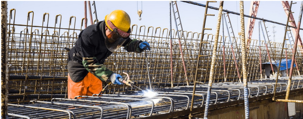
Fig. 5.16: Reinforcement fabrication with gas welding.
