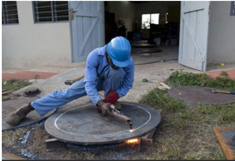
Fig. 5.22: Teaching gas welding school.
