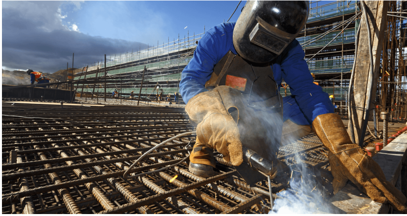
Fig. 5.24: Electric arc welding in the construction industry.
