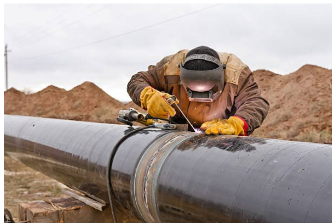
Fig. 5.26: Electric arc welding in Pipelines and Oil/Gas Industry.
