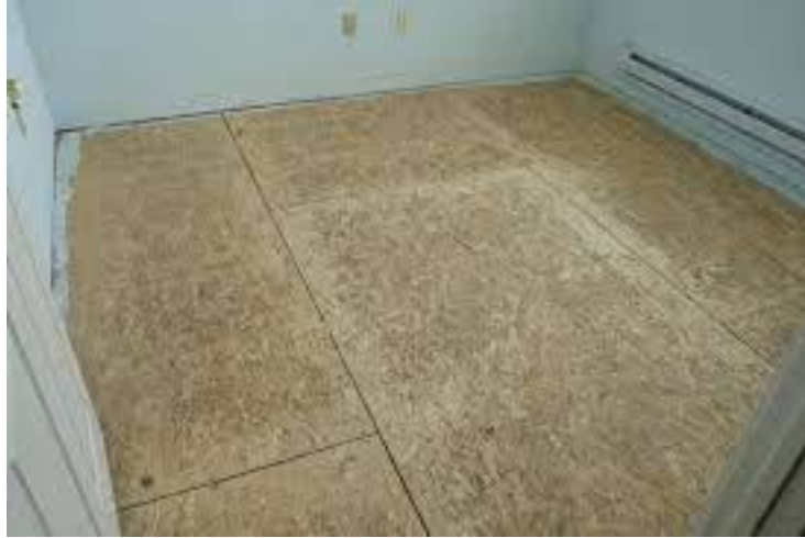
Fig 6.3: Oriented strand board in use
