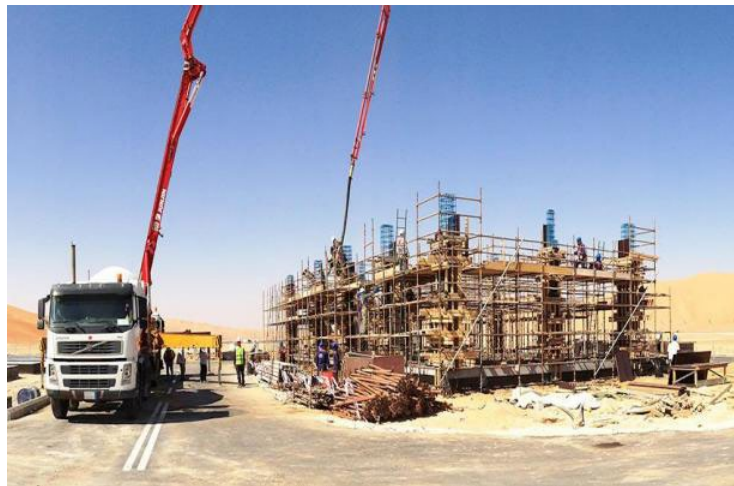
Fig. 6.14: Open space around the work zone to enable fire Service, hoists, and other plants access.
